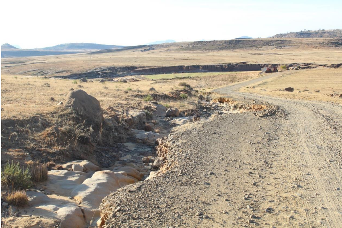
Figure 24: Erosion scars / gullies along the gravel road from Tsoloane Village to Thabana-Morena, Zone 6 (SEED, 2018)
